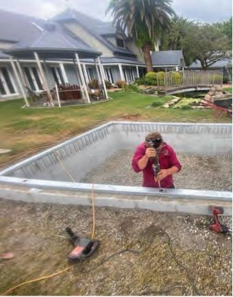
Tradesman in action bolting down the frame to the masonry walls of the pit.
