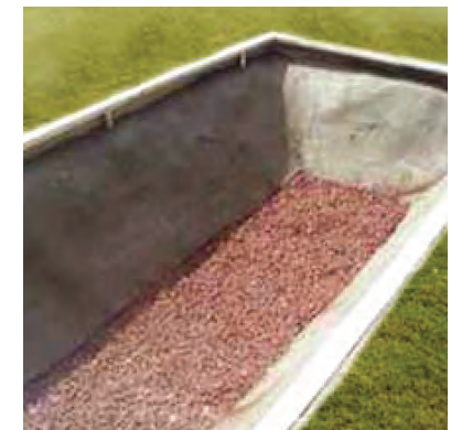
6. Clean out the pit
