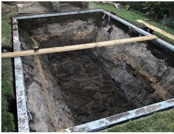
**Tips:** start from one end and work your way back. Pit recommended depth is 1200mm and should slope towards your pump (if you are installing one) or drainage pipe if you are choosing natural drainage. Please refer to IN GROUND TRAMPOLINE INSTALLATION PLAN AND SECTION drawings (specifically Pit detail section) for more accurate details
