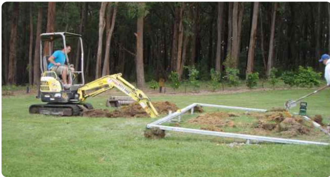
Excavating the pit, with the frame in place as the guide.
