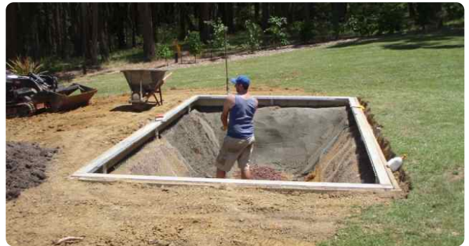
Finishing the render coat — the base falls gently to the drain.
