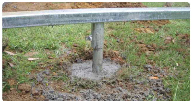
Each leg cemented into its footing with the frame held level.
