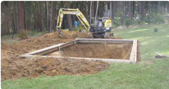
Working back from one end; spoil goes to the low side.
