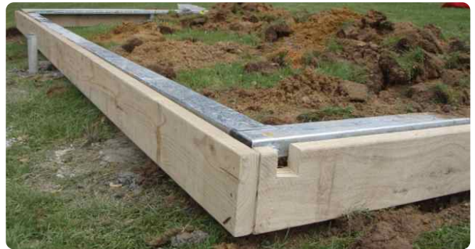
Sleeper retaining wall built hard against the frame to hold the built-up soil.
