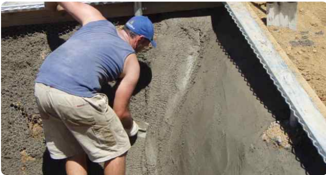
Rendering the pit walls over chicken wire.
