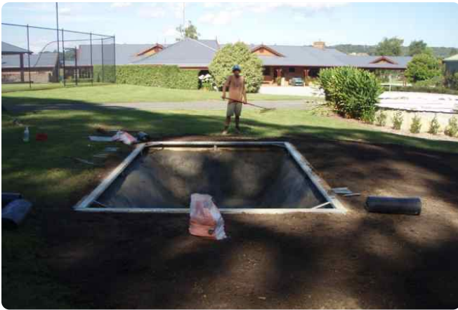
Finished pit, ready for the mat and springs.
