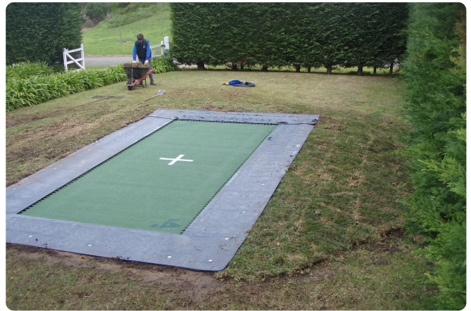
Finished trampoline, level and flush with the built-up lawn.
