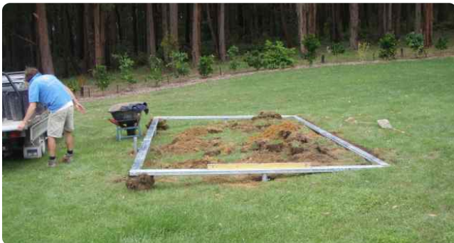
Bolt and square the frame first, then use it to mark each footing.
