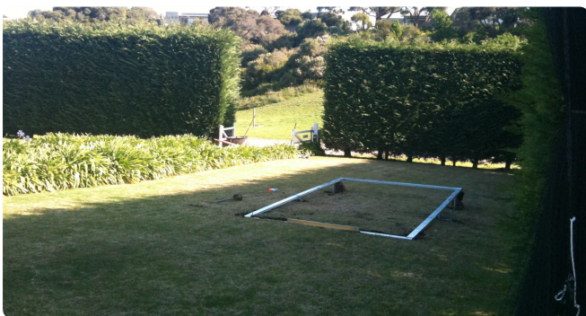
Frame set level across the slope — the low side is propped until the concrete sets.
