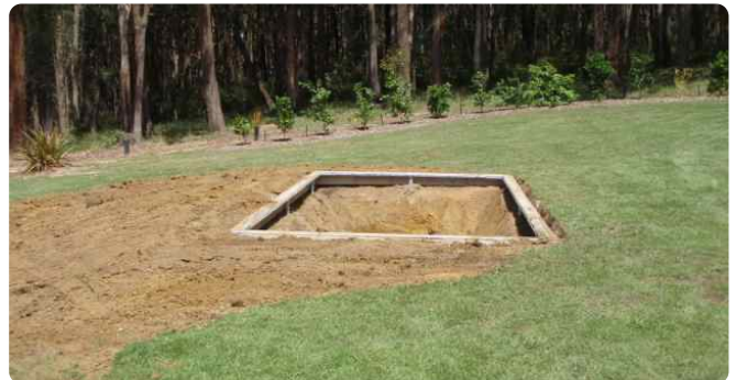
Pit excavated and the surrounding ground built up level with the frame.
