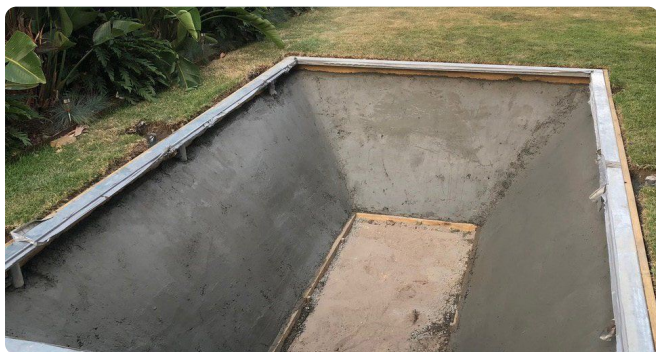
The rendered pit, ready for the mat and springs.
