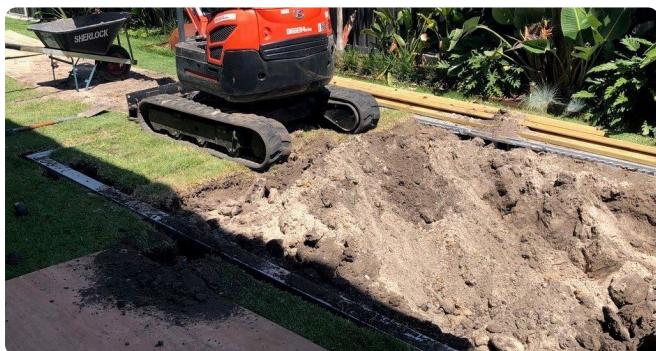
Digging the pit inside the assembled frame — a mini excavator makes short work of it.
