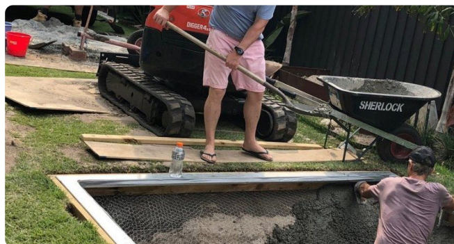
Rendering the pit walls over mesh gives a neat, long-lasting finish.
