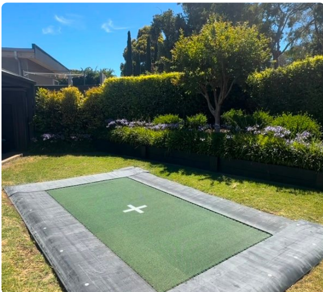
Done: rubber down, screws in a straight line, and the overhang settling onto the lawn.
