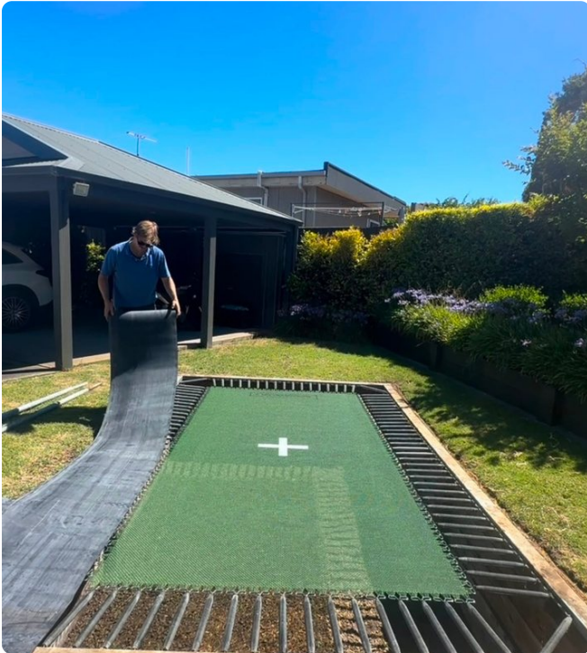
Unrolling the first long side along the frame — flipped over from the way it was rolled, so it lies flat.
